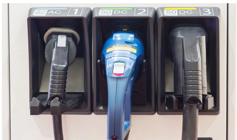
Figure 8. Charging Stations with AC, DC (CHAdemo) and DC (CCS) Connectors
